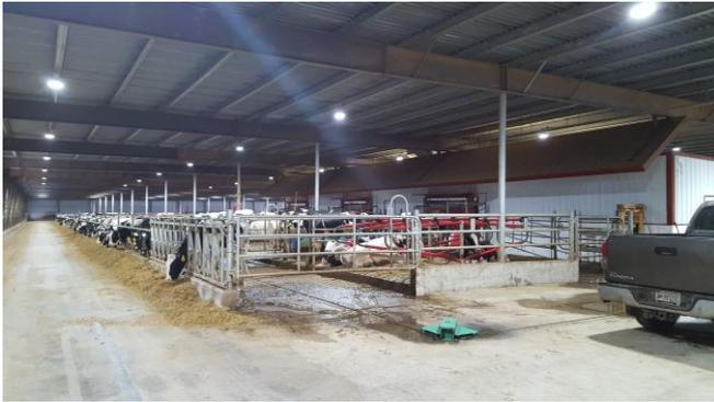
It comprised of 36 Lely Astronauts, each milking 60-70 cows, all under one roof. The herd was split into 12 sections, 3 robots in each serving 180-190 cows, with 2 sections (6 robots) for heifers. Central areas were used as extra handling facilities and dry cow and transition pens were also in the same facility. The whole building was mechanically ventilated, and cleanliness and hygiene were of the highest priority.
